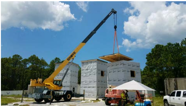
Temporary moisture protection added to cross-laminated timber (CLT) blast testing structures.
